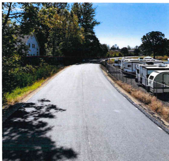
Molalla Forest Rd. has been reconstructed and widened to accommodate modern traffic to Chief Yelkus Park and the Bear Creek Subdivision from Toliver Rd.
