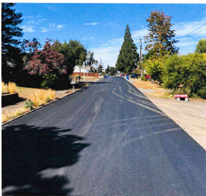
6th St. has been grind & inlayed with minor widening
