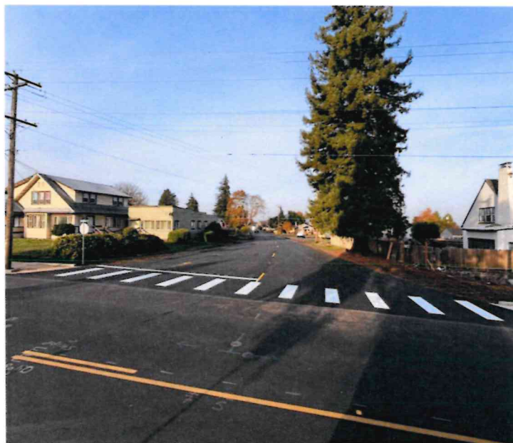
Section St. has been fully reconstructed to correct geotechnical deficiencies and is a vital part of the downtown bypass trucking route.
