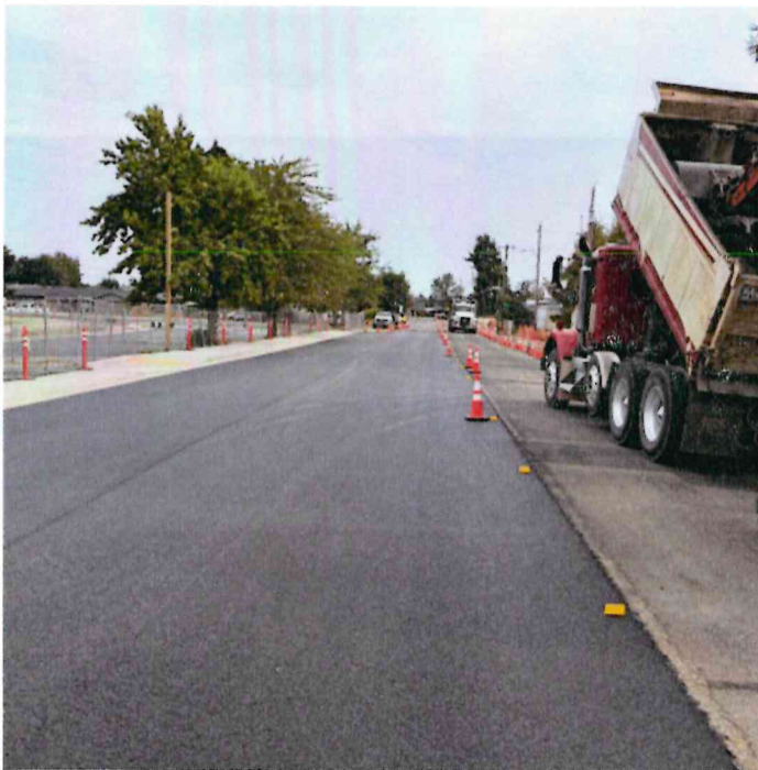
Widening and paving of Leroy Ave. related to the Molalla River Middle School construction project. The full street to Toliver, as well as Lynn, Hezzie, and West Ln. is actively permitted.
