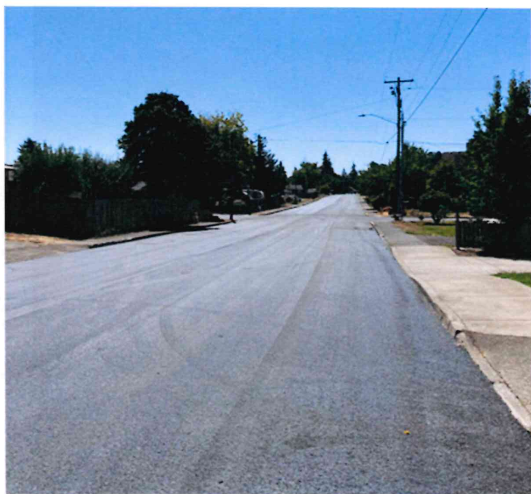
Paving on N. Cole Ave. to Main St., extending up to and including Frances St. to N. Molalla Ave.
