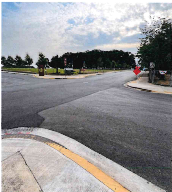
Grind & Inlay street restoration of N. Cole Ave. and Shirley St.
