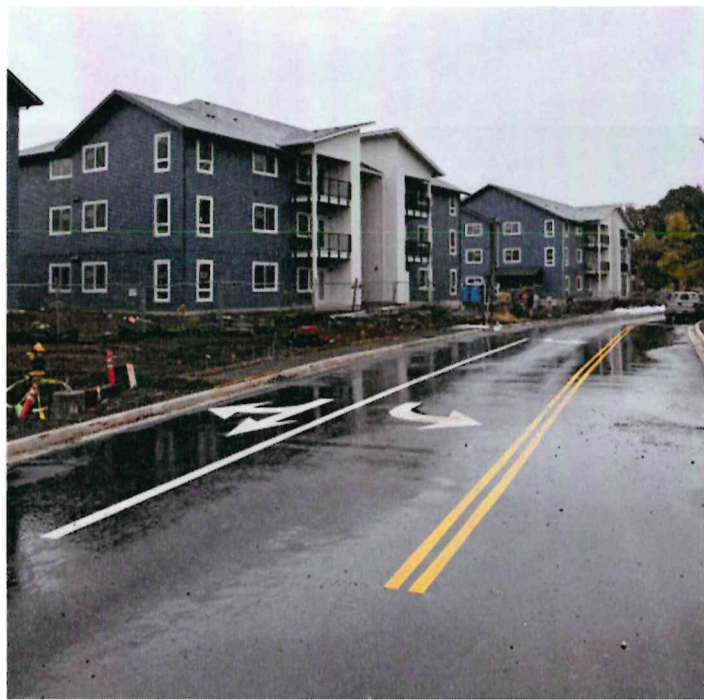
S. Ona Ln full street improvements completed related to the Bear Creek Apartments Ph.II construction project. Additional work on HWY211 conditioned by the City allowed for current active construction of N. Ona Ln to the Bear Creek Subdivision
