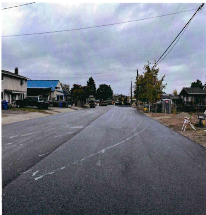
Lola Avenue utility and street reconstruction
