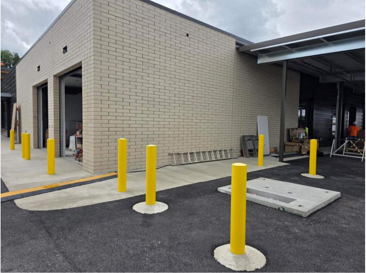
Figure 2- 8.7.2025- PGE transformer pad and bollards
