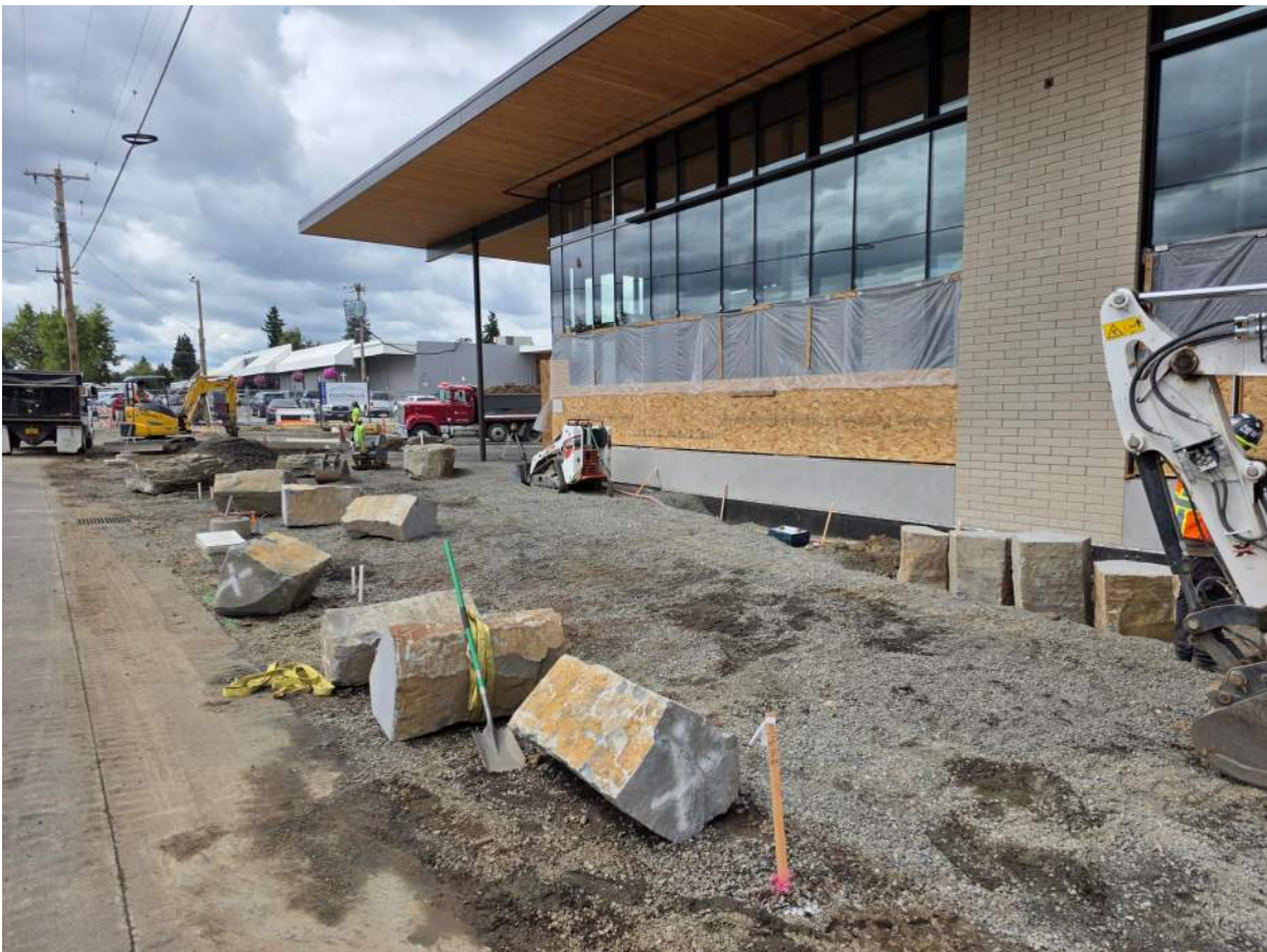
Figure 1- 8.7.2025- Basalt columns at sidewalk laid out
