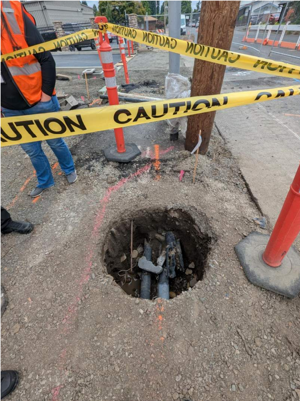
Figure 9- 6.26.2025- Unknown MCC conduit under light pole bases at entry ROW
