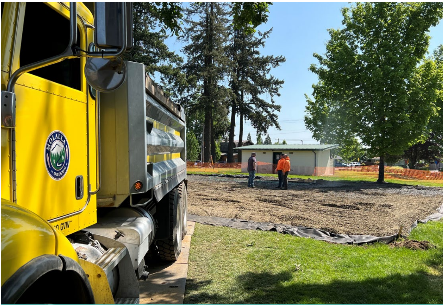
Long Park pickleball court construction
