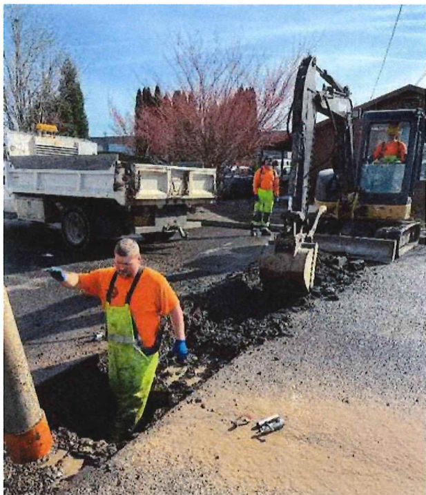
L: PUBLIC WORKS CREW IS REPLACING A WATER SERVICE ON CENTER STREET.
