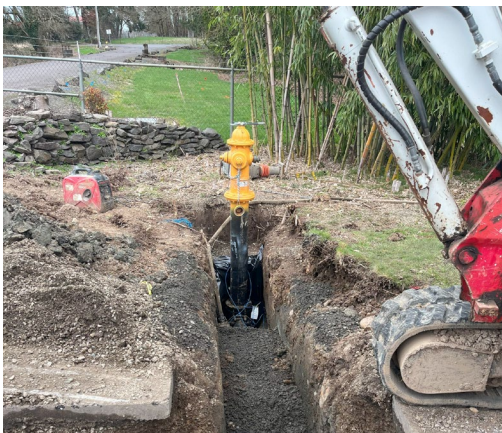
Installed new fire hydrant
