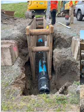
14" Transfer Line and 18" effluent discharge line
