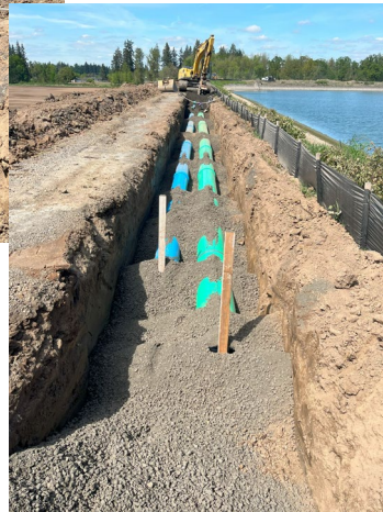
14" Transfer Line and 18" effluent discharge line
