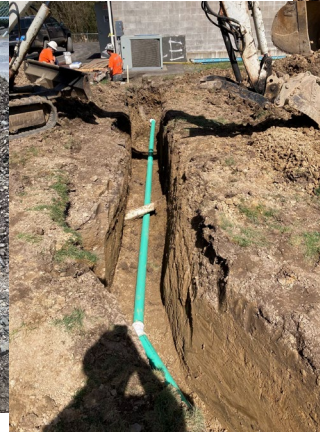
Re-routed a small in plant lift station
