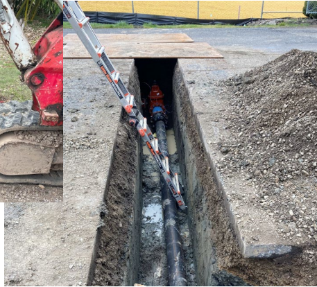
14" Transfer Line and 18" effluent discharge line
