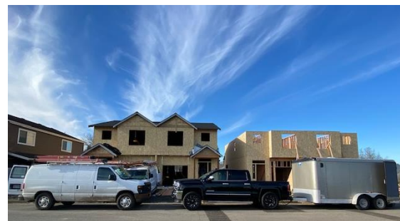
2 New Duplex's under construction on Eckard Dr.
