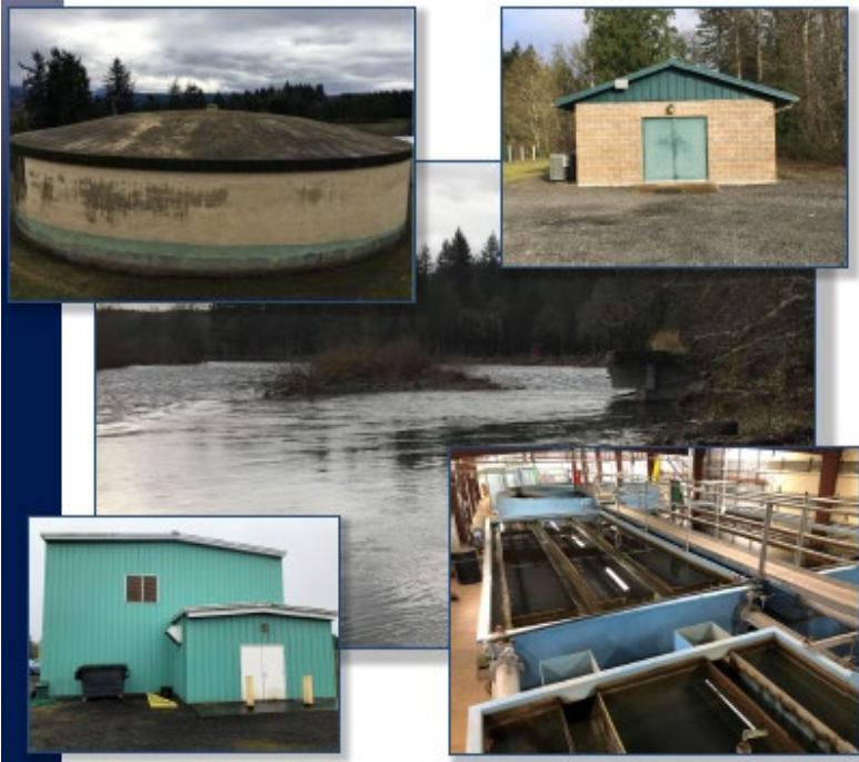
Various Pictures of Molalla's Water Treatment Plant
