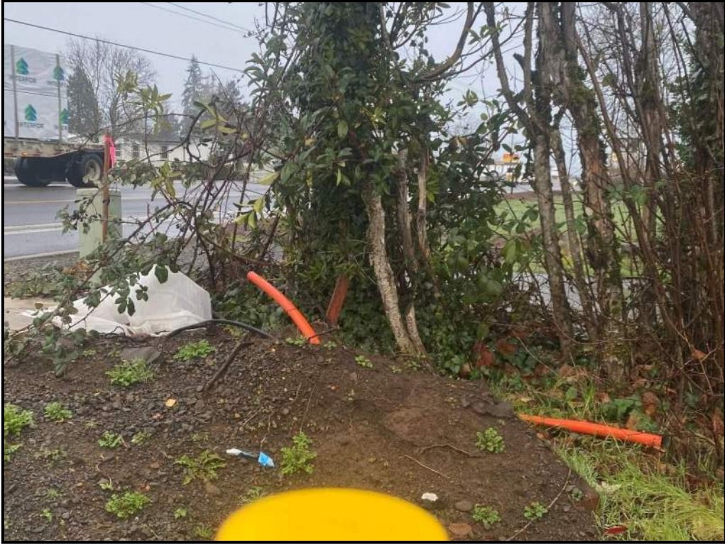
Figure 1: Site Access Looking East- 15' From Edge of Travel Lane
