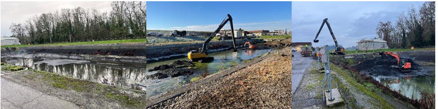
Aeration Basin Cleanout
