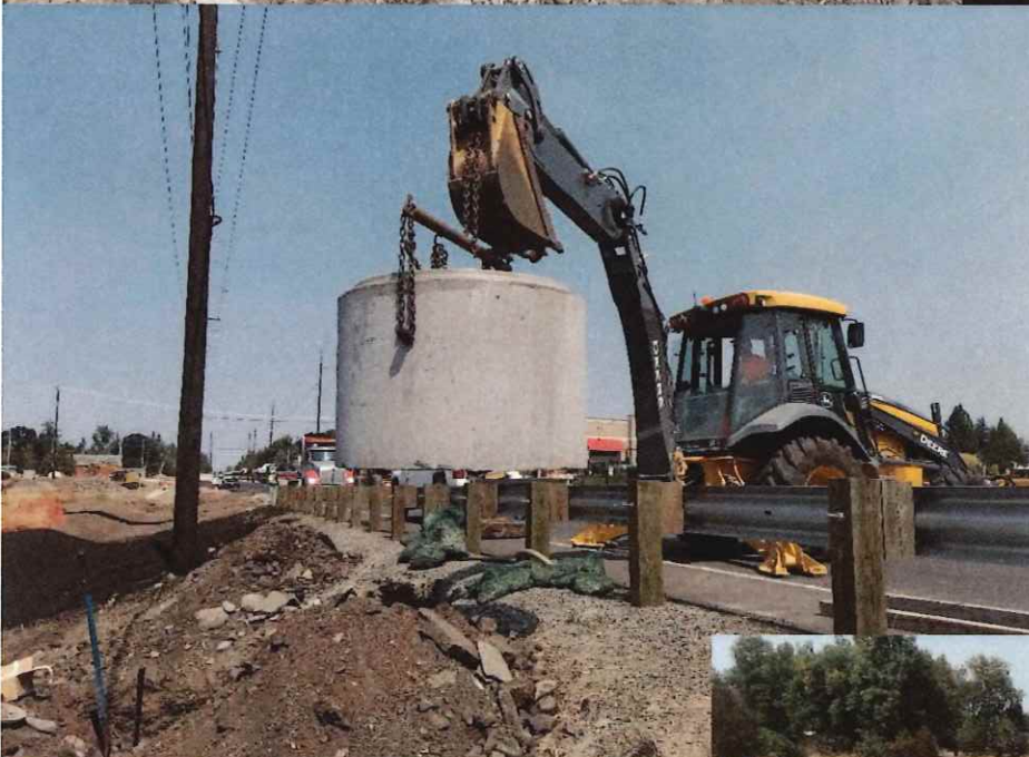
Public Works Utility Crew Adding a Section on Manhole to the Sewer Main on Hwy 213 during the Roundabout Project
