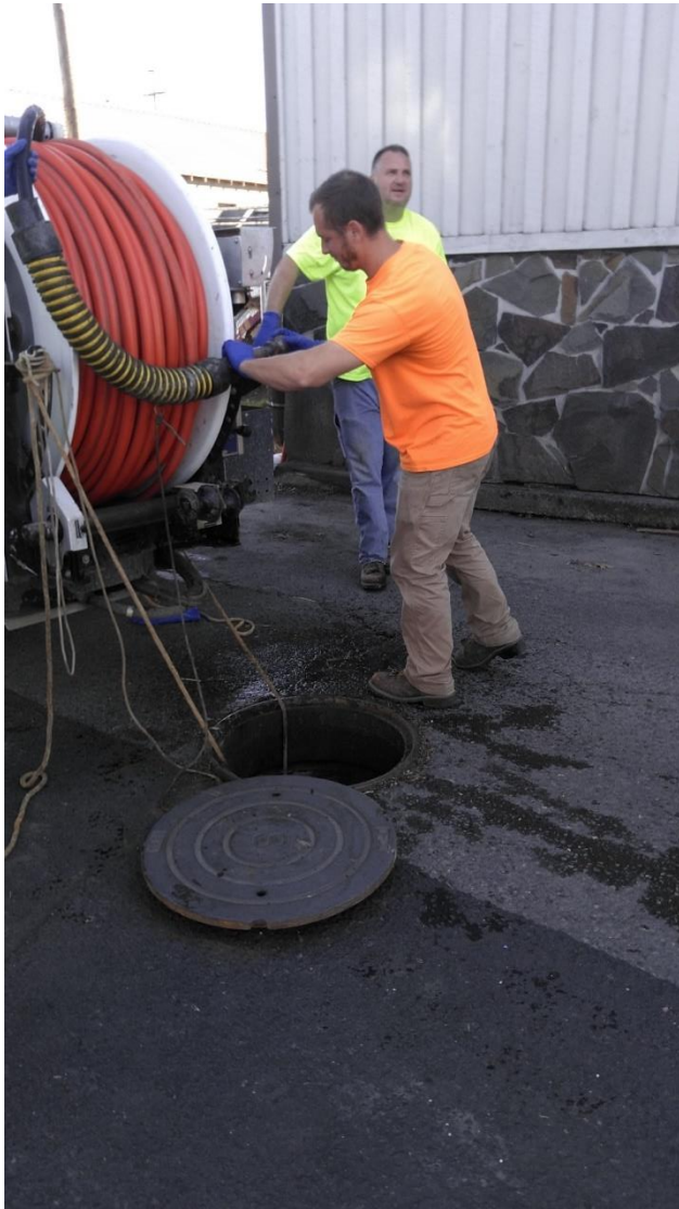
Sewer line cleaning and inspections were performed this month. Left, Cody and Shawn set up the vector to hydro jet public mains. Below, Cody inspects the grease trap at a local restaurant.
