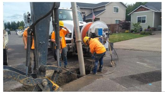
Left and below, City crews continue to repair water services in Big Meadow. New reporting capabilities put in place by the City shows a regular water loss in the system of roughly 30%, which is high. There are several factors contributing to this loss in addition to simple leaking services. For example, high mainline pressures. These have been addressed in the recent Water System Master Plan with pressure reducing strategies that will be achieved on upcoming capital projects.
