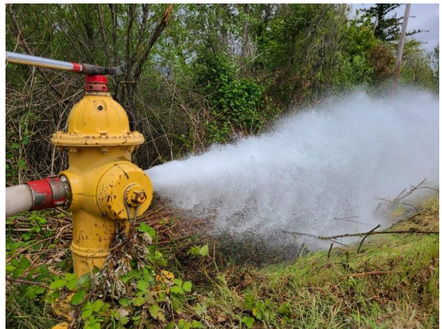
Right: Spring Flushing and Hydrant Exercising
