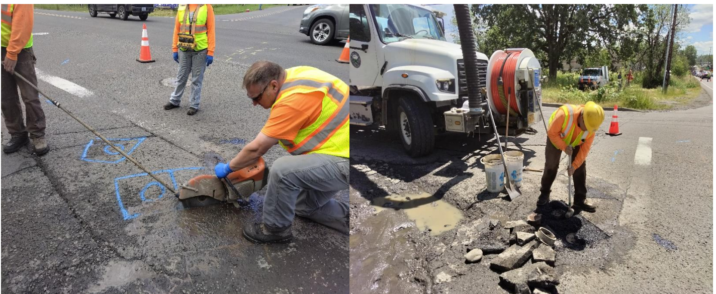
Below: Public Works utility crew uncovering buried water valves on Hwy 213.
