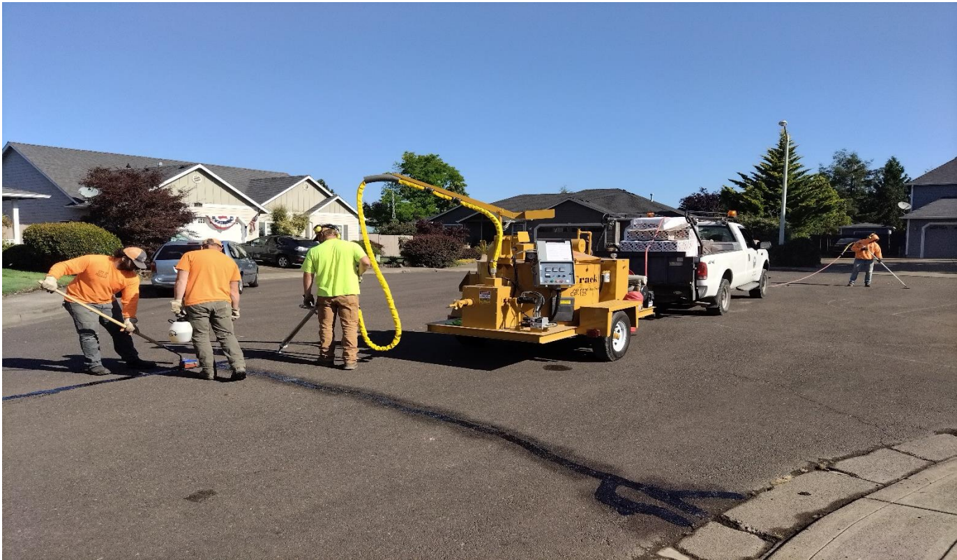
Utility crew crack sealed 1.3 lane miles applying 2250 lbs of sealent. This should add 5 to 10 years to the asphalt life.
