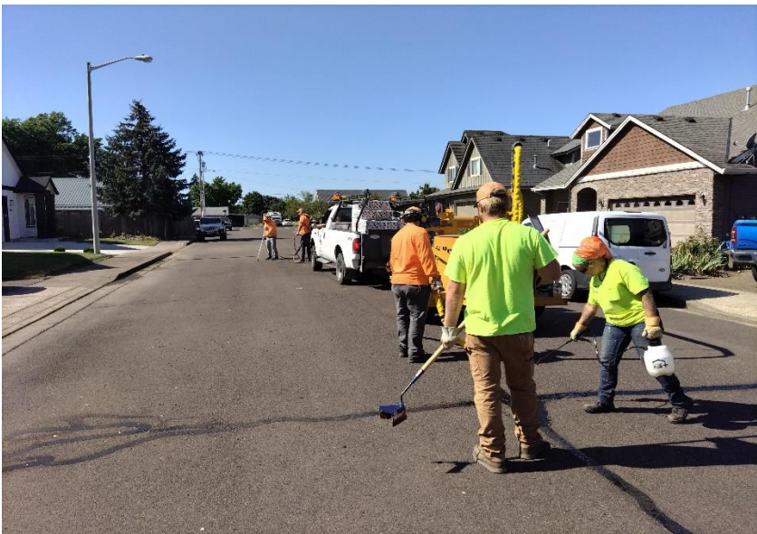
Utility crew crack sealed 1.3 lane miles applying 2250 lbs of sealent. This should add 5 to 10 years to the asphalt life.
