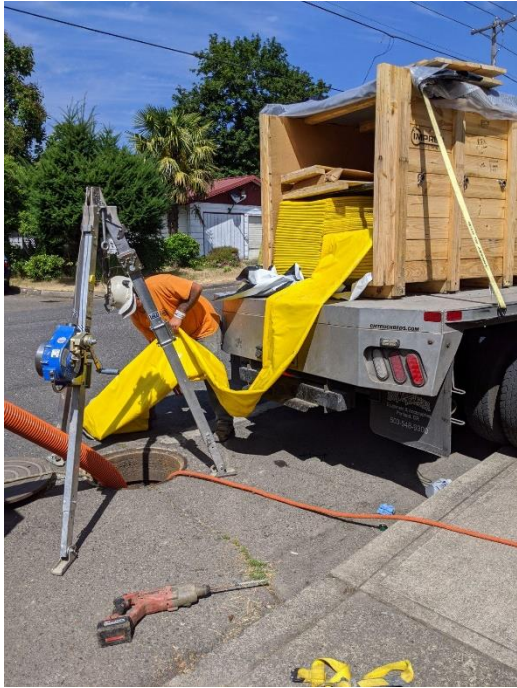
Above: Lining a section of Toliver sewer main with cured-in-place pipe.
