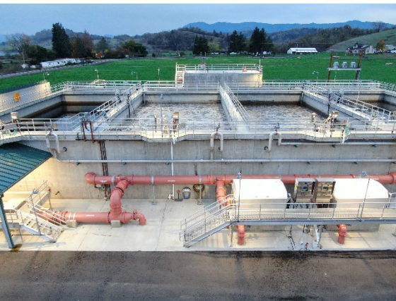
An example of the SBR type Wastewater Treatment Plant that will be built in Molalla, in part with Sewer SDC's
