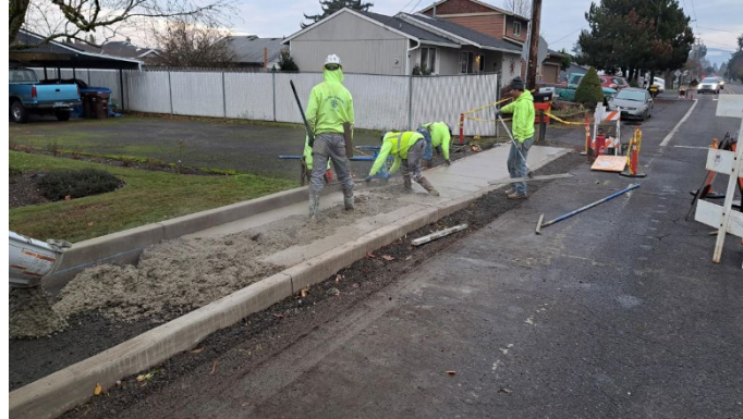
Sidewalk Infill in conjunction with an Emergency Water Main Repair on Toliver at N Leroy Ave
