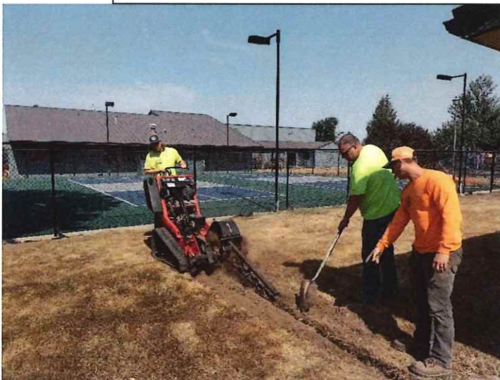
Utility Crew installing the signage and irrigation at Long Park for the Pickleball Courts
