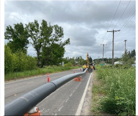
HDPE Pipe to be installed Under Bear Creek Culvert
