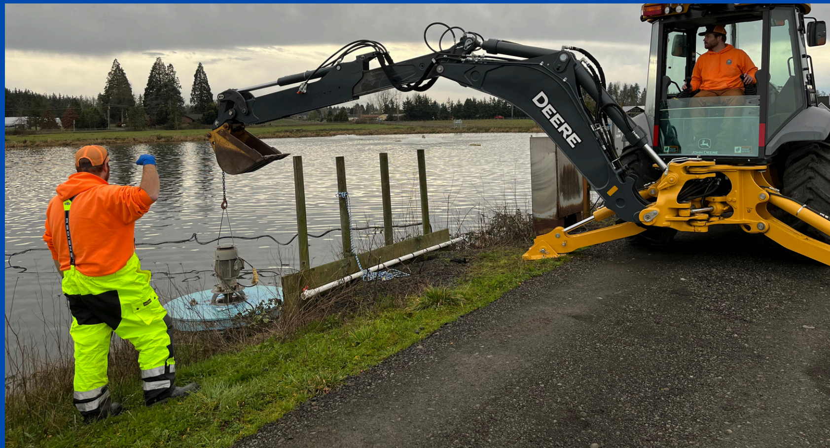
Aerator Maintenance at the Wastewater Plant treatment lagoons
