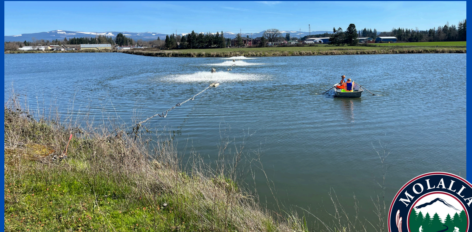
Aerator Maintenance at the Wastewater Plant treatment lagoons
