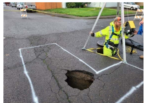
Crews repair a Sink Hole in Big Meadow
