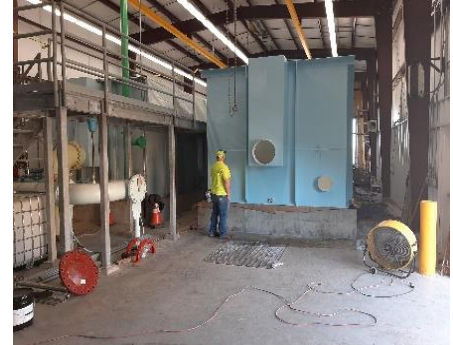
Molalla's Water Treatment Plant Operator Admires the New
