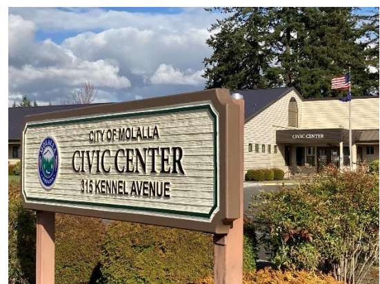
The newly established Molalla Civic Center provides office space, Council Chambers, and the Municipal Court room
