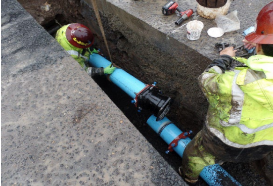
A New Water Main is Installed in the 500 block of W Main St. – Water loss was reduced by 15% this Fiscal Year!
