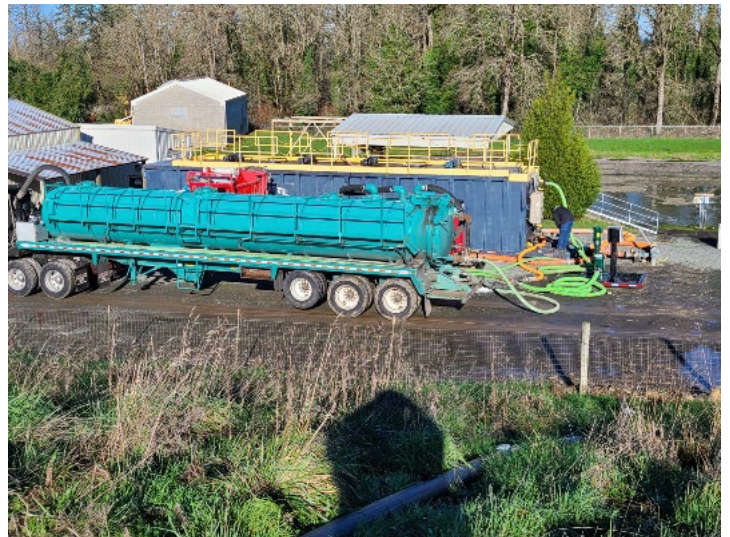
Biosolids Removal is now a continuous operation at Molalla's Wastewater Treatment Plant
