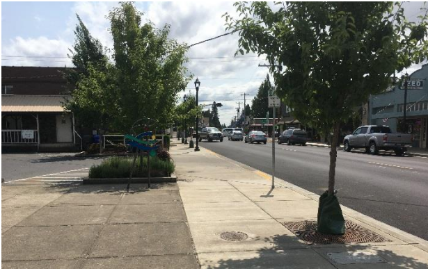
Improved Sidewalk on Molalla Avenue
