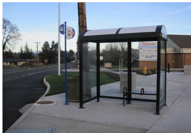
TriMet Stop (After)
