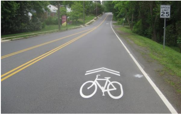
Example of Shared Lane Pavement Marking (Sharrow)
