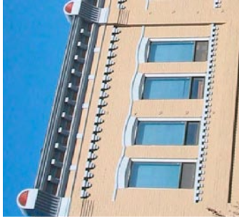
Windows with unified lintels and sills
