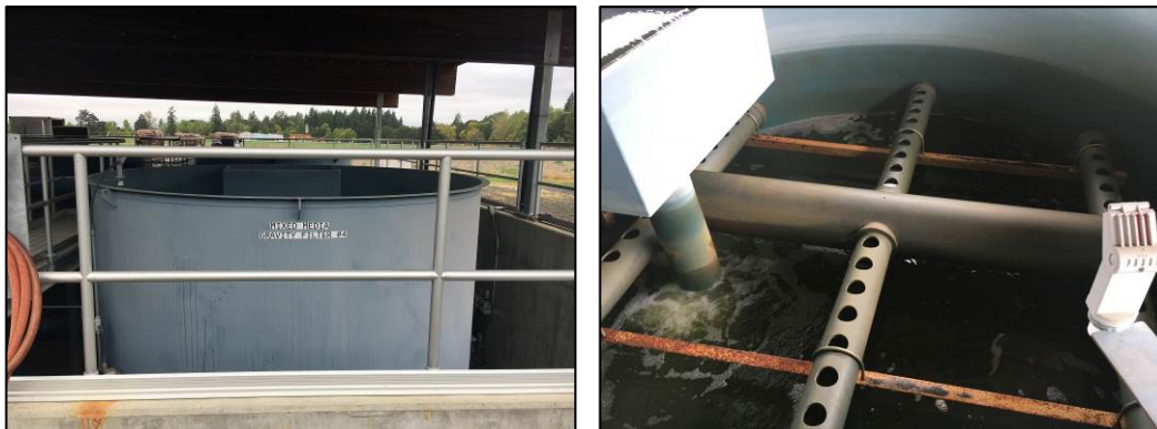
FIGURE 2.3.24 GRAVITY FILTERS
