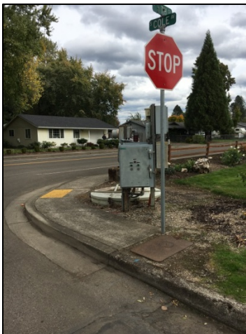
FIGURE 2.3.10 EAST 5 TH AND SOUTH COLE PUMP STATION
