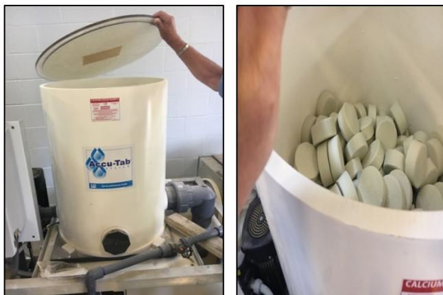
FIGURE 2.3.25 TABLET CHLORINATION
