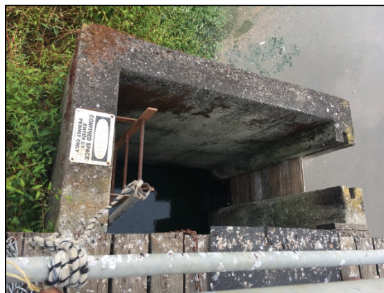
FIGURE 2.3.19 LEVEL CONTROL STRUCTURE
