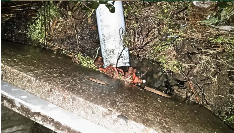
Site map of Spill (above), image of broken service line (left).
