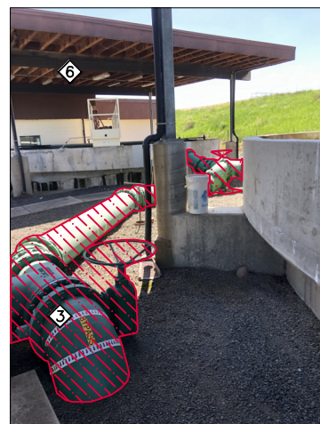
PHOTO: EXISTING DAF PIPING
