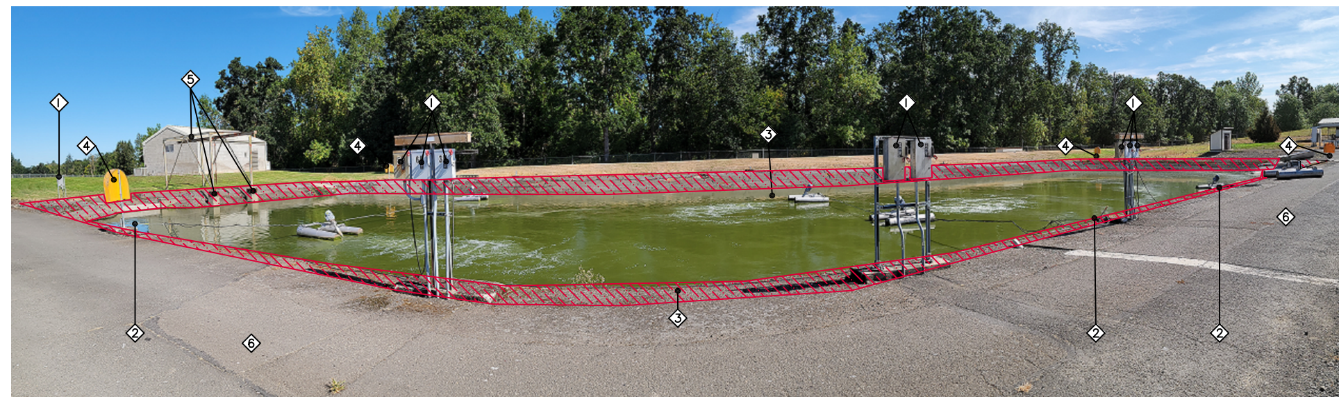
PHOTO: AERATION BASIN - DEMO COMPONENTS A
