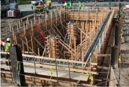
Cast In Place Concrete Forming
