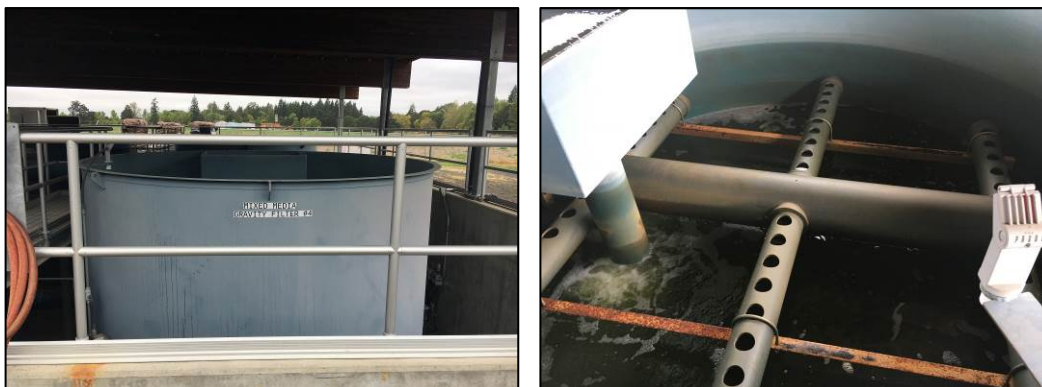
FIGURE 2.3.24 GRAVITY FILTERS
