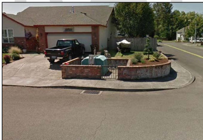
FIGURE 2.3.9 TAURUS PUMP STATION
