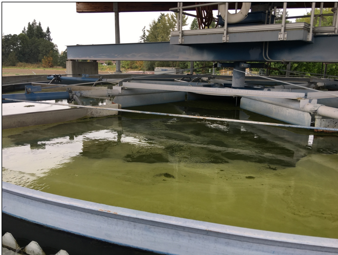
Figure 3-5: Flotation Thickener Process
