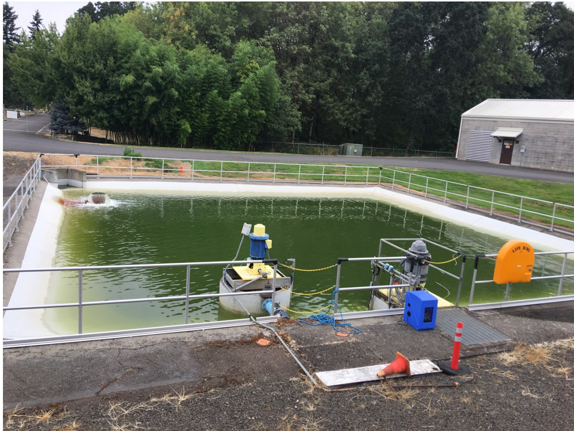
Figure 3-6: Algae in Chlorine Contact Tank
