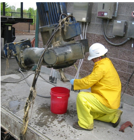
Operators take sewage pumps out of service and use hand tools to remove clogs.
