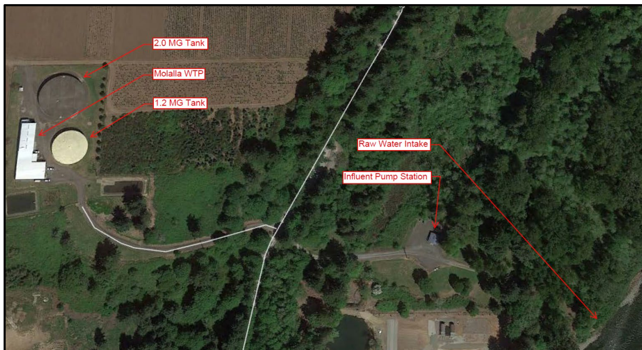
FIGURE 5.3.1 WTP EXISTING SITE
